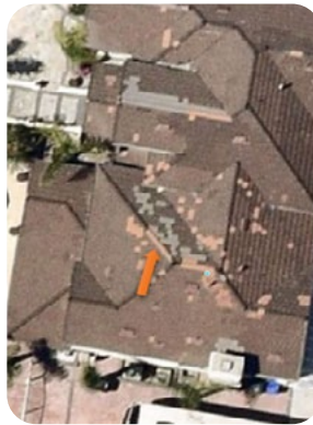
Missing Shingles
